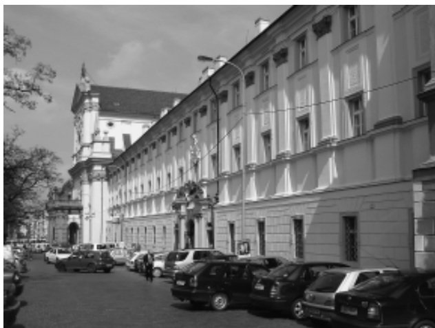
Figure 2 – The central part of main building with the Church of St. Ignatius, where is now situated the Third Clinic of Internal Medicine of the General Teaching Hospital and the First Faculty of Medicine of the Charles University in Prague.
